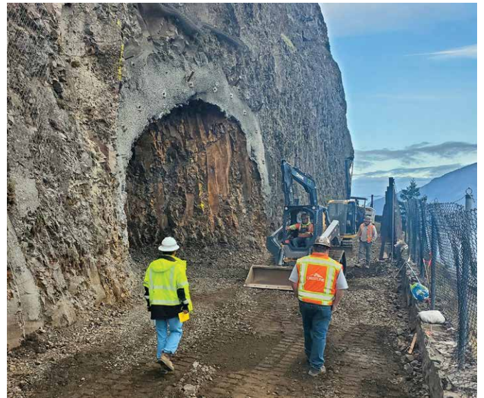
Crews excavating the tunnel entrance at Mitchell Point.
