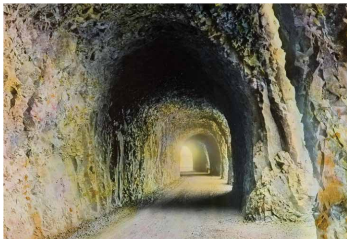
Light streamed into the original Mitchell Tunnel through river-facing “windows.” Photo: Courtesy of Oregon Department of Transportation
