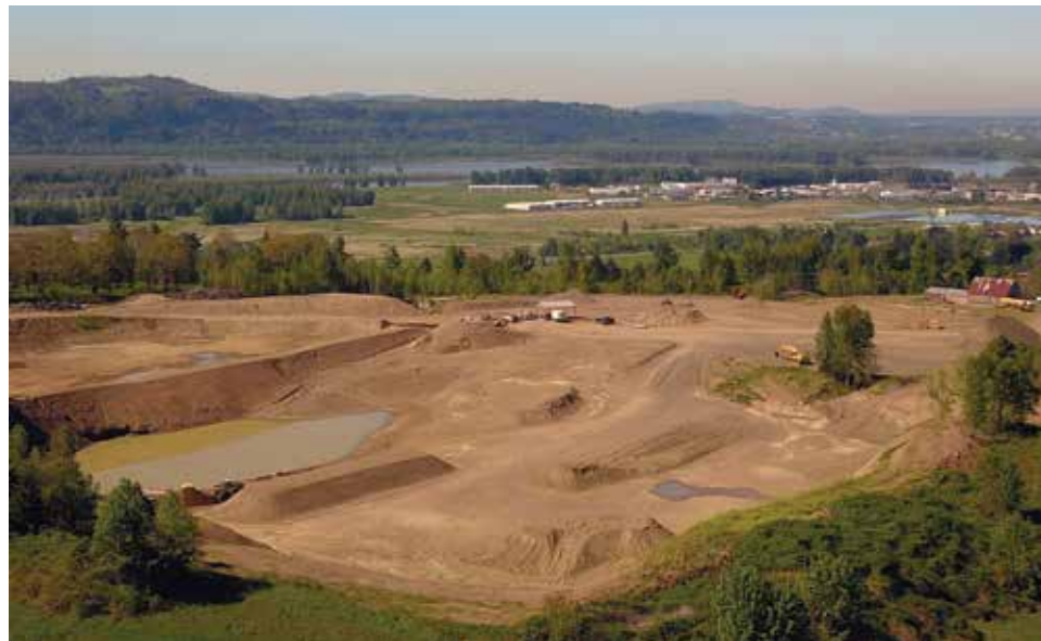
This unpermitted quarry operation lies inside the National Scenic Area near Washougal, Washington.
