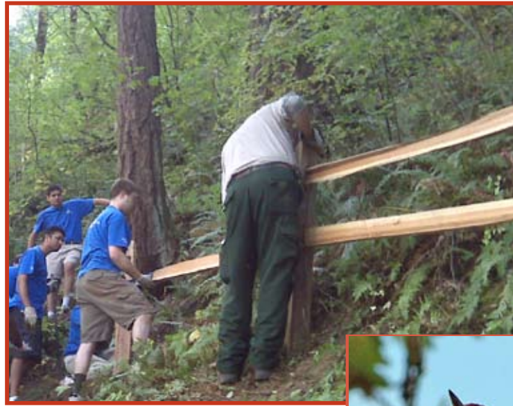
Volunteers building fencing along the Multnomah Falls switchback.
