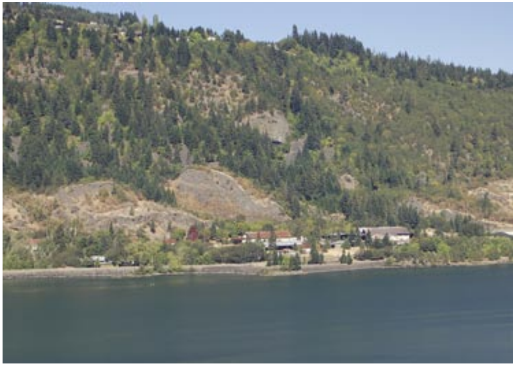
Broughton Lumber Company is proposing a 260-unit destination resort on this site in the Columbia River Gorge National Scenic Area. Photo: Aubrey Russell
