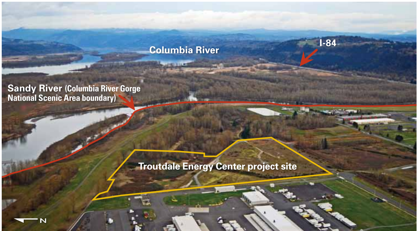
The project site for the now-abandoned Troutdale Energy Center lies just a few hundred feet from the western bank of the Sandy River, which is also the boundary of the Columbia River Gorge National Scenic Area. Photo: Rick Till; map labeling: Kathy Fors
