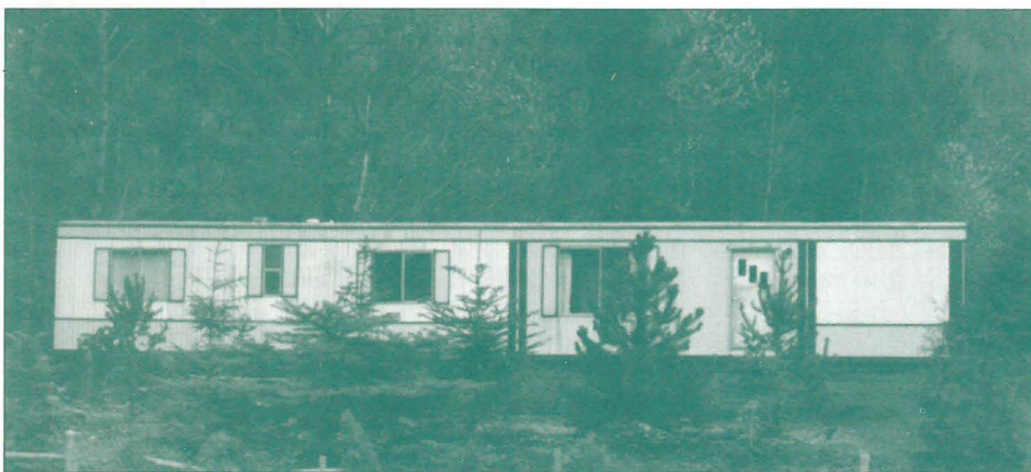
Mobile homes have no permanent foundations and can be removed easily. A new Gorge Commission policy, challenged by FOCG, would allow any mobile home in the Gorge to be replaced with a permanent, site-built home.
